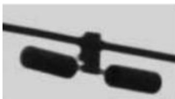
(b) 防震锤 (b) Vibration damper
